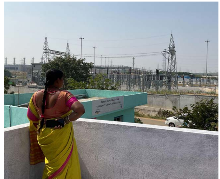
AWS Data Center in Begarikancha
